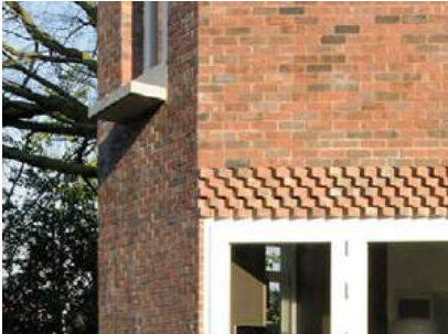
BRICK DETAILING ADDS TEXTURE AND INTEREST
