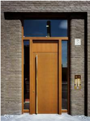
LEGIBLE ENTRANCE TO APARTMENTS USING TACTILE MATERIALS
