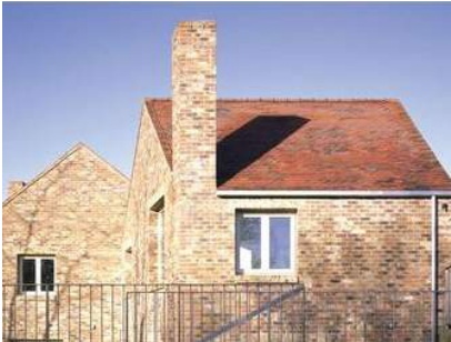
PRINCIPAL MATERIAL TAKEN THROUGH ENTIRE BUILDING
