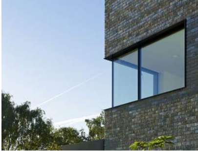
RECESSED CORNER WINDOW WITH SLENDER FRAME SECTION
