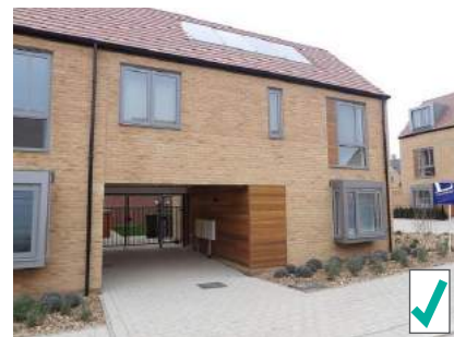
UNOBTRUSIVE SERVICES BOXES IN A PARKING ZONE
