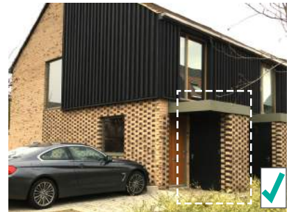
SERVICES CONCEALED IN EXTERNAL CUPBOARD
