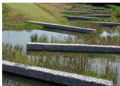
DETENTION BASIN BAFFLES
