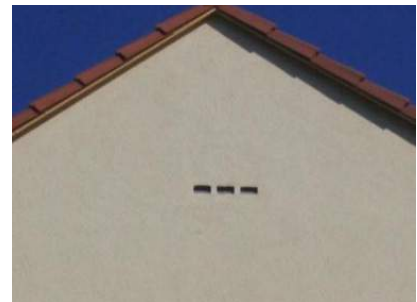
INSTALLED BAT TUBES (X3) WITH A RENDERED FINISH (SOURCE: THE BAT CONSERVATION TRUST WEBSITE)
