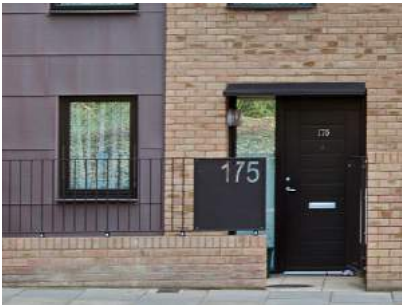
EXAMPLE OF AN INTEGRATED BIN STORE WITHIN THE BOUNDARY OF A PRIVATE ENTRANCE
