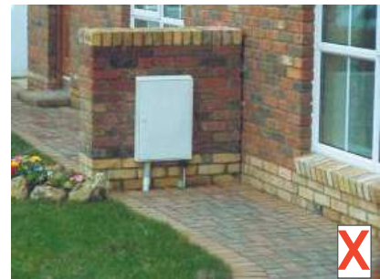
OBTRUSIVE SERVICES BOXES ON FRONT ELEVATION
