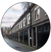
CAR PARKING AT REAR IN GARAGE WITH ACCOMMODATION ABOVE (P.23)
