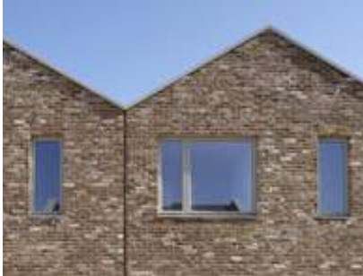
WELL ORDERED FLUSH COMPOSITE WINDOWS
