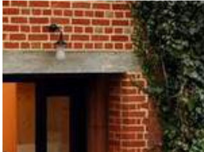
CONCRETE LINTELS ABOVE DOORWAYS
