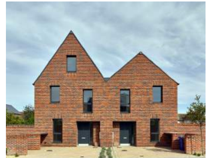
VARIED ROOF PITCHES ON A PAIR OF SEMI-DETACHED HOUSES
